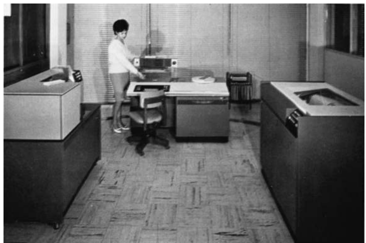
Figure 2. The first IBM 1130 at Aereofoto, circa 1966. At this early installation, temperature was controlled with an air-conditioning unit mounted on a window while cables were initially exposed. (Courtesy of Fundación ICA.)
