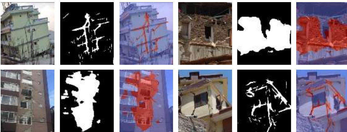
Figure 10. Some examples of correct prediction for cracks and spalling by cascaded networks (cracks and spalling are in red and white for the overlaid and predicted images, respectively, and background of the predicted images is in black).
