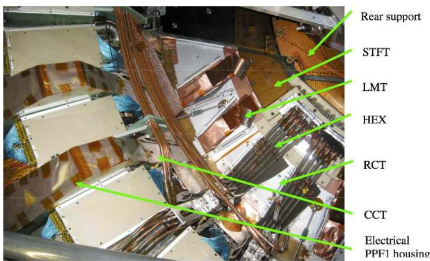
Figure 56. View of services, in particular the cooling circuits and the LMTs, at the rear of the end-cap and inside the cryostat. At this stage, the feed-through boxes were yet to be added to seal the STFT and the rear sections of the RCT are not in place.
