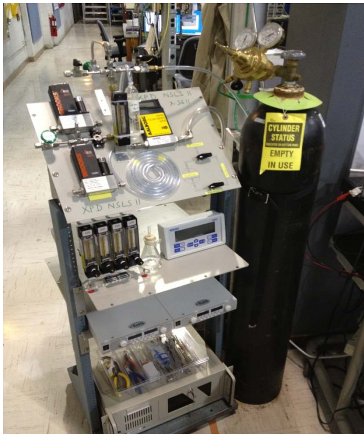
Figure 8. New automatic gas manifold and temperature controller designed and assembled at NSLS, BNL.
