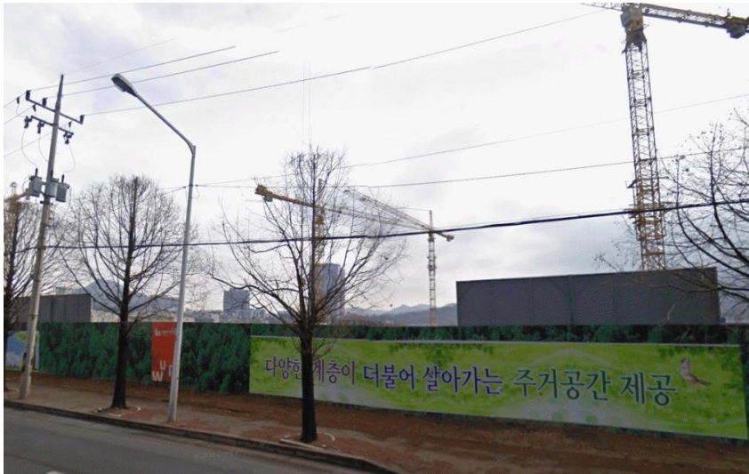
Figure 2. Forestwood under construction
