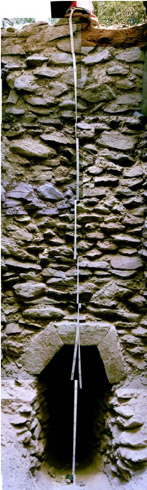
FIGURE 6. Combined elevation photo of the northern wall of the subterranean water system under the cubicles in the Azāzo residence, with the entrance to the subterranean water tunnel; 2011 excavation. Photo by the Universidad Complutense Ethiopian Jesuit Missions Project.
