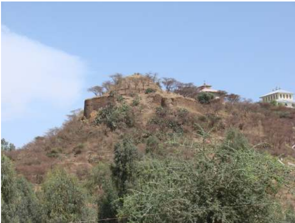
FIGURE 38. The remains of the defensive walls and bastions of the Jesuit Mission of Fremona, Tigray. At right, the new churches of St. George and St. Abuna Aregawi. The big earthen mound beneath the walls was possibly formed by the many recent graves excavated in this Orthodox holy place. Photo by V.M. Fernández.
