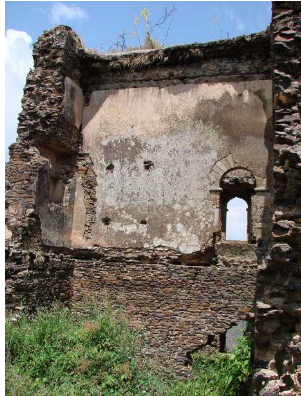
FIGURE 26. One of the best preserved walls of the Dänqäz palace, with the plastered wall and an arched window of the residential second floor. Photo by V.M. Fernández.
