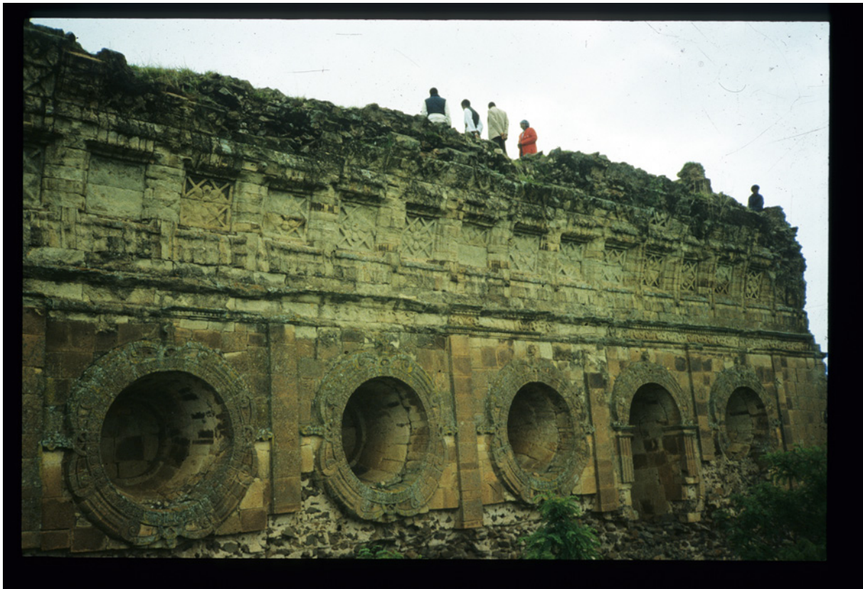
FIGURE 16. The southern wall of the Gorgora Nova main nave. Decorative blind windows ( oculi ) were disposed all along the wall. Photo by J. González Núñez (1986). Reproduced with permission.
