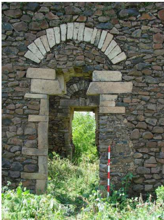
FIGURE 23. One of the arched doors of the Däbsan Jesuit residence. Photo by V.M. Fernández.
