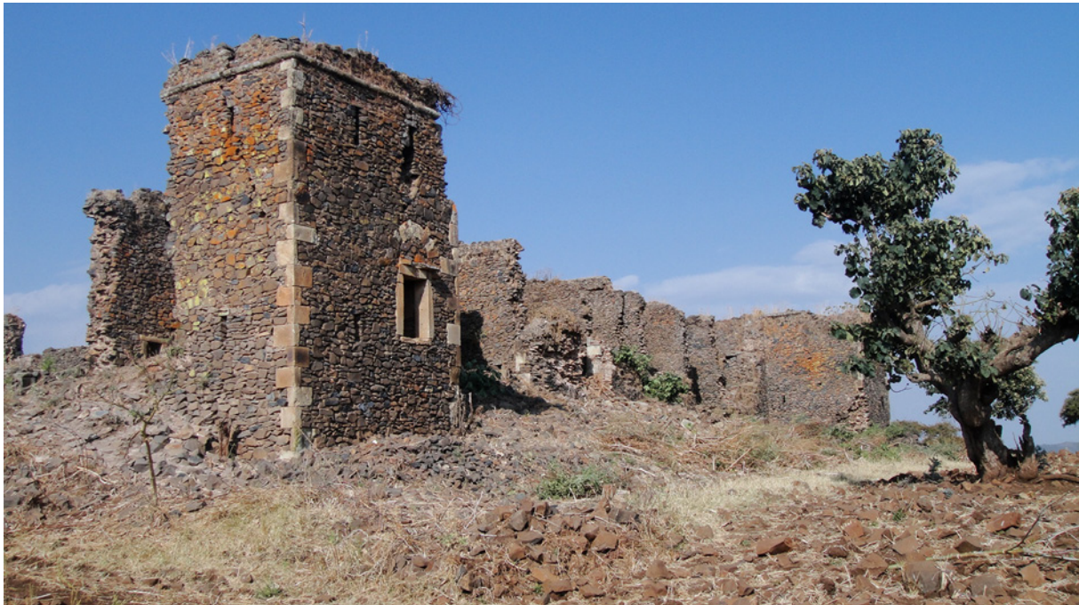
FIGURE 19. Lateral view of the Gorgora Nova residence with the western tower in the foreground. Photo by V.M. Fernández.
