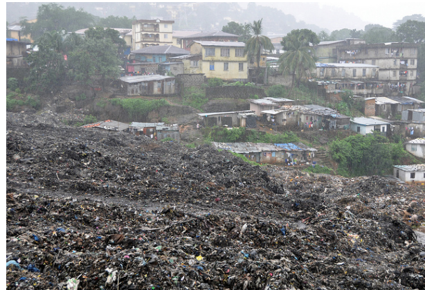
Figure 1. Granville Brook dumpsite overlapping residential houses at Racecourse Culvert slum.
