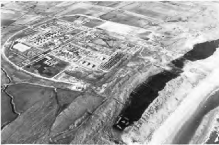
Photo 2. A general view of the St. Fergus terminal and adjacent coastline at an early stage of site work.
