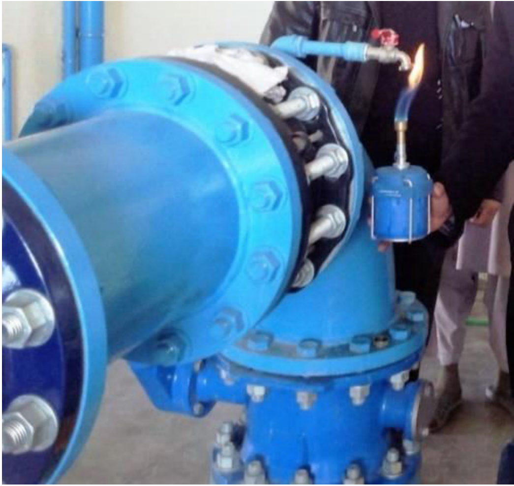
Fig.3.4: Heat sterilization of a water supply booster pump by a gas torch before sampling
