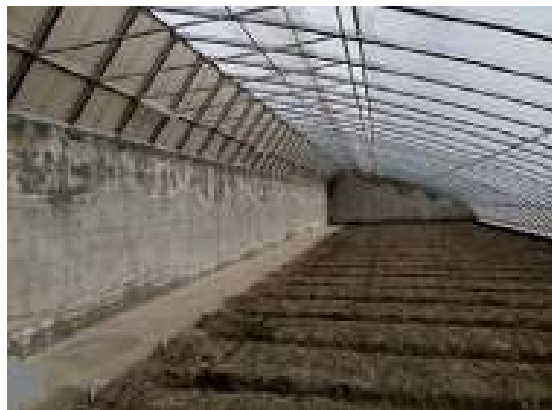
Figure 1. Clay Chinese greenhouse north wall [1].
