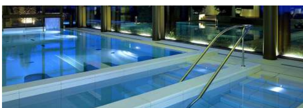
Figure 3: Advanced solutions permitted by bended tiles as stairs, walls or swimming pools
