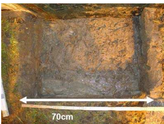
Figure 5.19 Length of the prepared hole.
