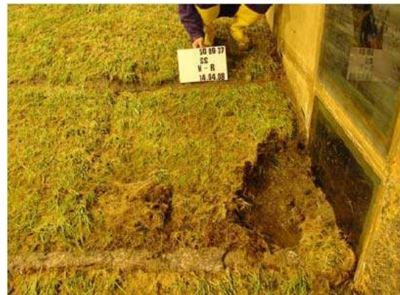
Figure 5.15 First damage on the observation window (after impact).
