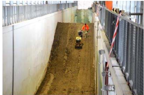
Figure 3.13 Clay compaction with a roller.
