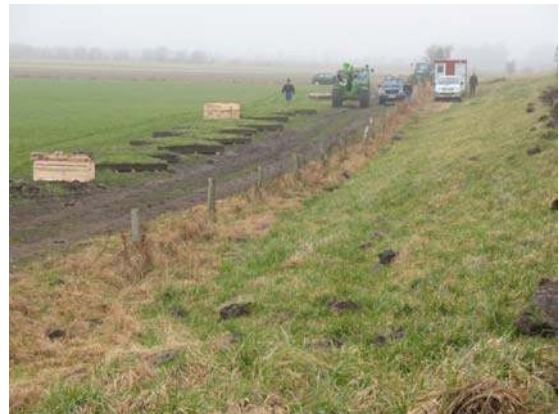
Figure 3.17 Temporary storage of the excavated grass sods on an adjacent field.
