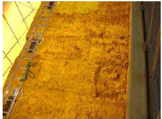
Figure 5.24 Degradation of the grass cover in the breaker zone.
