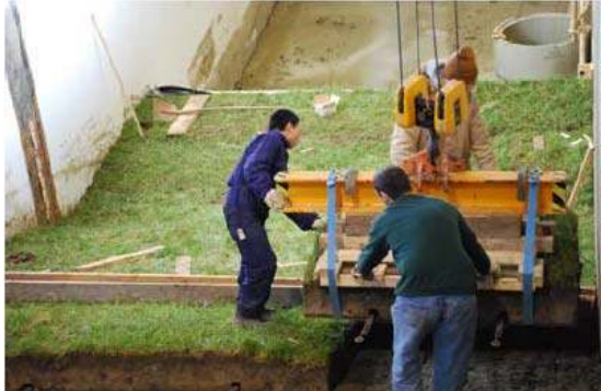
Figure 3.28 Installation of the third grass sod of a row.
