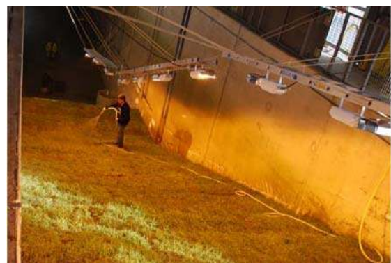
Figure 3.43 Irrigation of landward slope.
