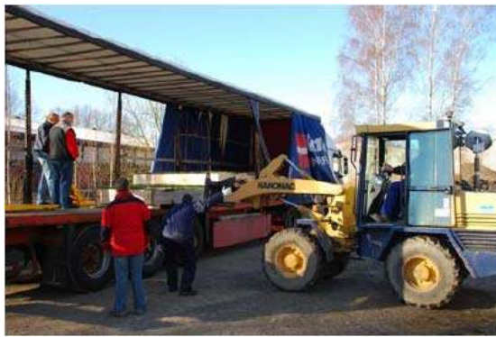
Figure 3.20 Unloading of the grass sods at the Coastal research Centre in Hannover.
