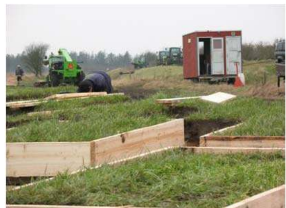
Figure 3.19 Construction of wooden frames around each grass sod.
