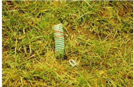
Figure 4.4 Empty cladding tube including the pull rope inside.
