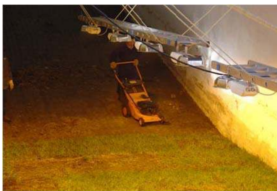
Figure 3.42 Mowing the grass cover on the seaward slope.
