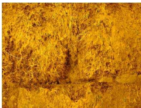
Figure 5.29 Damaged joint on the seaward slope during wave overtopping tests.
