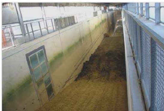
Figure 3.4 Final foreshore with clay depot for the seaward clay revetment.
