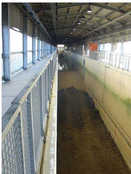
Figure 3.7 Simultaneous construction of the seaward clay layer on the dike model.
