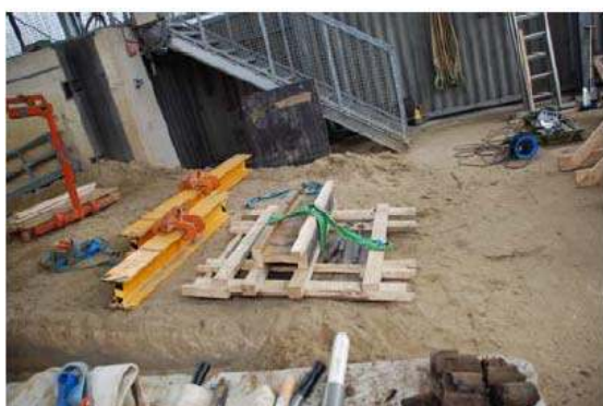
Figure 3.26 Wooden transport frame, steel hooks and two steel beams.
