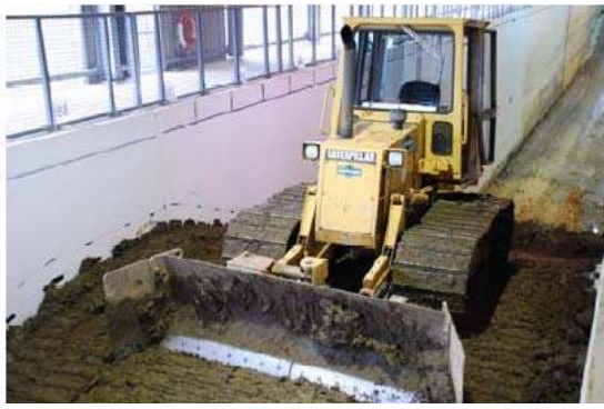
Figure 3.12 Loader used in the Large wave Flume.
