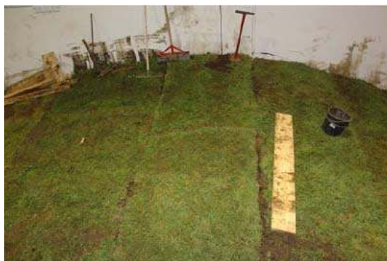
Figure 3.35 Dike crest with grass cover.
