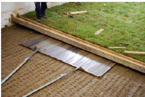
Figure 3.34 Pulling the underlying wooden plate.
