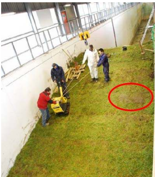
Figure 3.36 Compaction of grass layer on seaward slope.
