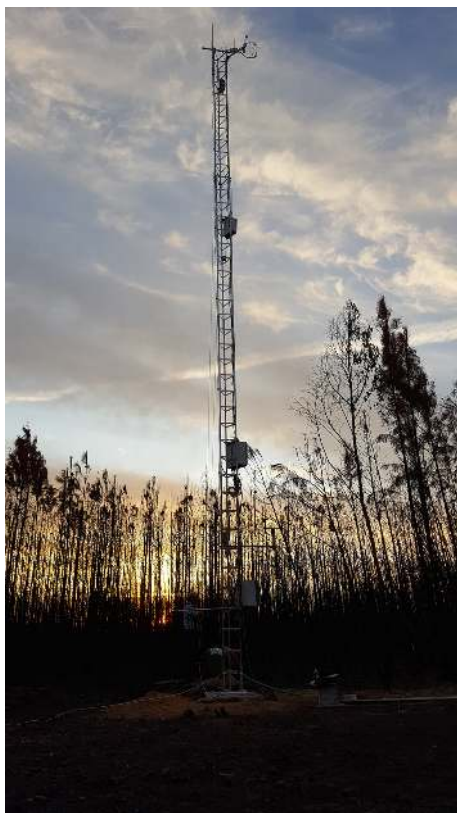
Figure 4. The 12 m slim tower with the eddy-covariance system immediately after its installation (photograph: J. Jacob Keizer, 22 September 2017).
