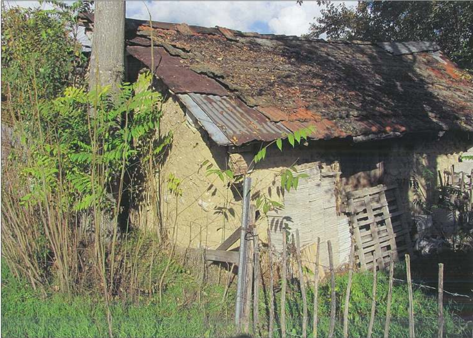
Figure 5. Northern building along Via San Nicola (photograph by G. Shaffer).
