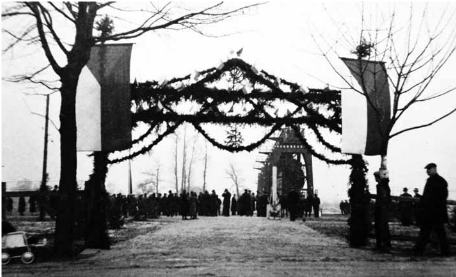
Figure 2.9 – In 1937, Czechoslovakia opened a new weir on the river Oder by Koblov. The hydraulic structure was hailed as a first step towards realization of the DOE. The ceremony was a national event with all the important figures in the Czechoslovak water engineering community attending, including Smrček and Bartovský. Source: ATMB, Smrček, b. 134.
