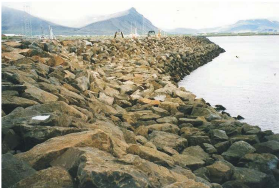
Fig. 6.7: Icelandic Berm breakwater
