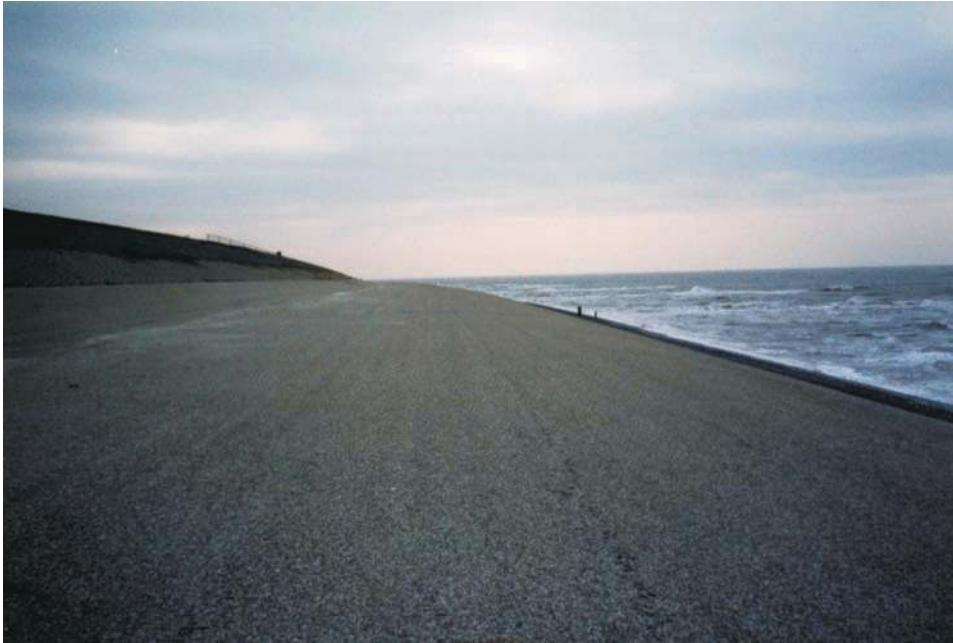
Fig. 5.16: Dike covered by asphalt (photo: SCHÜTTRUMPF)
