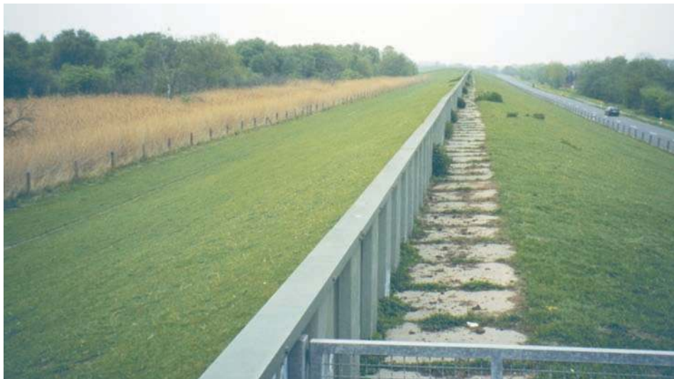
Fig. 5.30: Sea dike with vertical crest wall (photo: HOFSTEDE)
