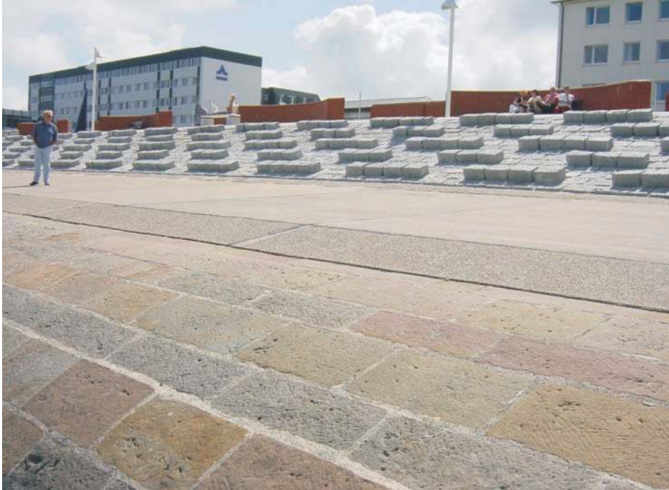
Fig. 5.19: Example for roughness elements (photo: SCHÜTTRUMPF)
