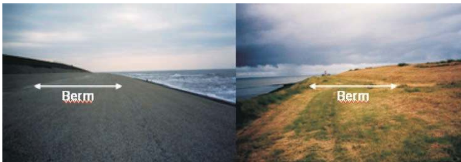
Fig. 5.28: Typical berms (photo: SCHÜTTRUMPF)
