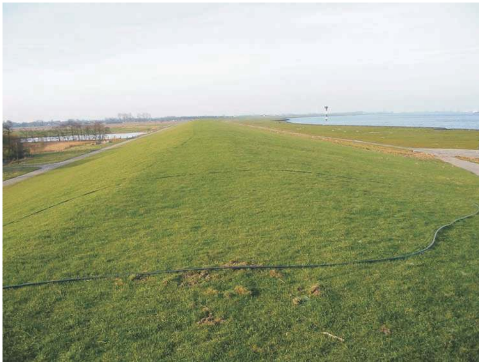
Fig. 5.15: Dike covered by grass (photo: SCHÜTTRUMPF)
