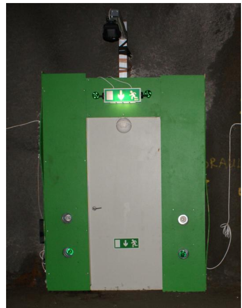
Figure 4. A picture of the emergency exit inside the tunnel.
