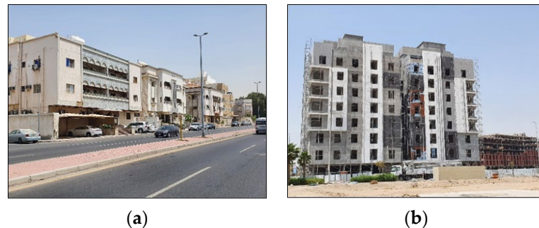
Figure 6. Differences between the old high-density zoning code and the new code: (a) old multistory building in Jeddah; (b) new multistory building in Jeddah.
