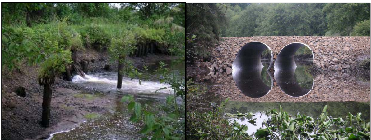
Figure 2.5. Tidegate at Kandoll Farm before (left) and Culverts after (right) Replacement
