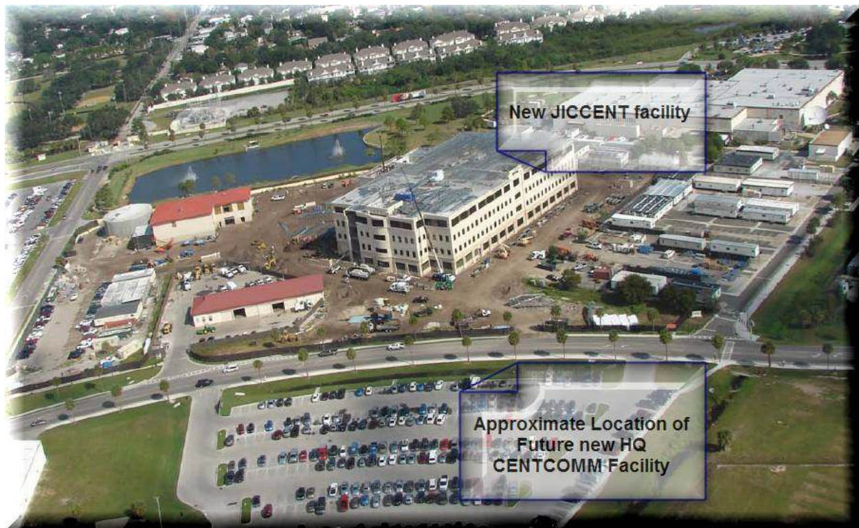
Figure 2-35. New JICCEN facility and future HQ CENTCOMM facility location on MacDill Air Force Base, Florida (Beam 2008)
