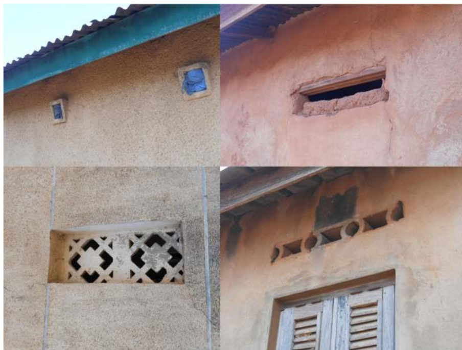
Fig. 3 Examples of ventilation bricks commonly found in the study area in central Côte d'Ivoire. These are often either left unscreened, or blocked (e.g. with LLINs, as shown in the top left image)
