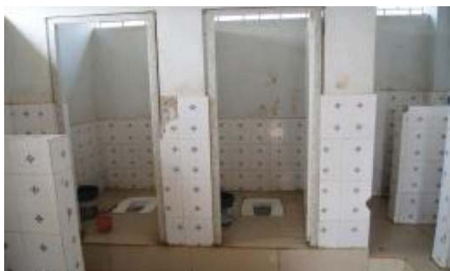
Figure S2. Girl's restrooms installed in a government high school.
