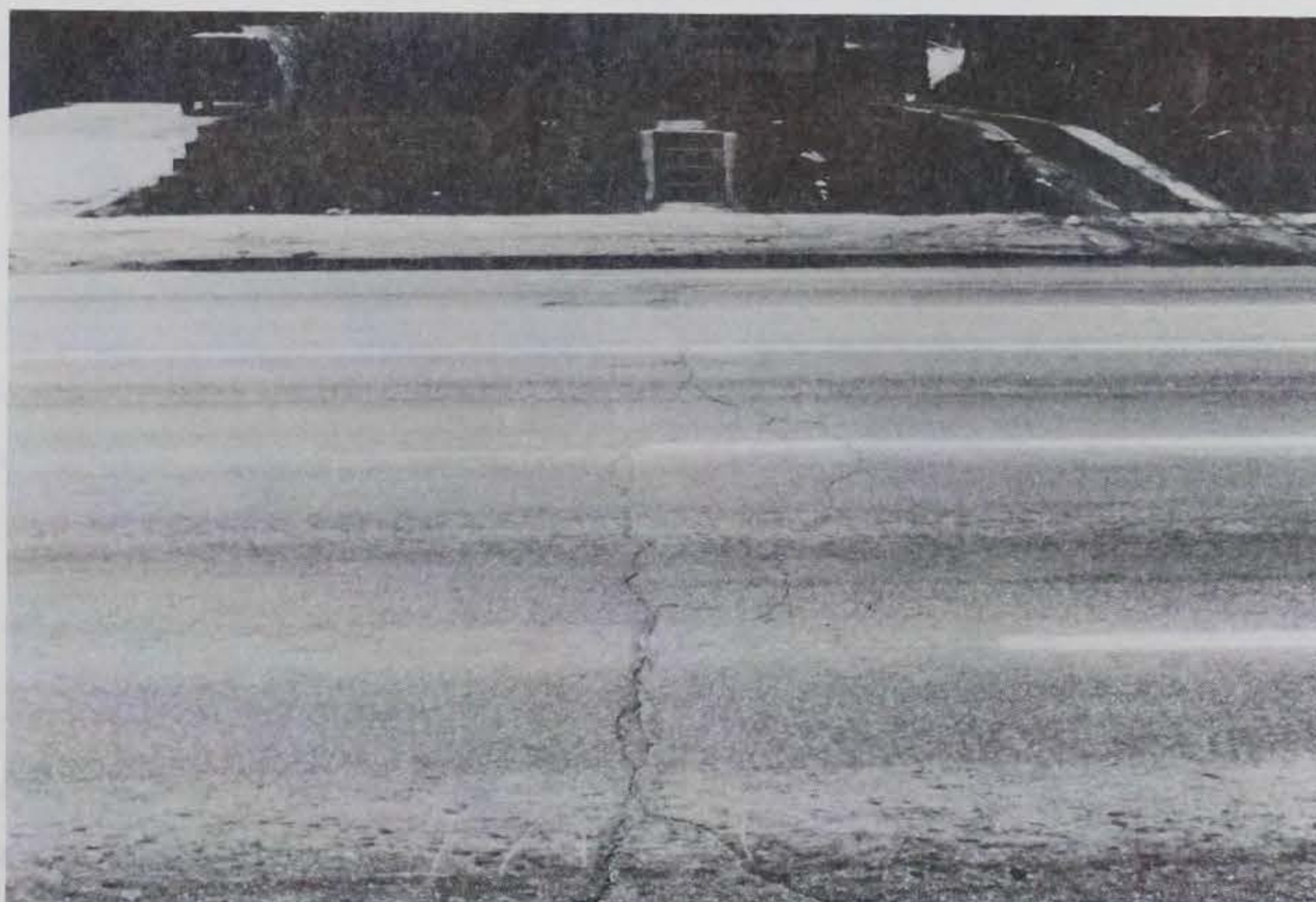
Figure 19. Engineering fabric section, Alameda Avenue, Denver
