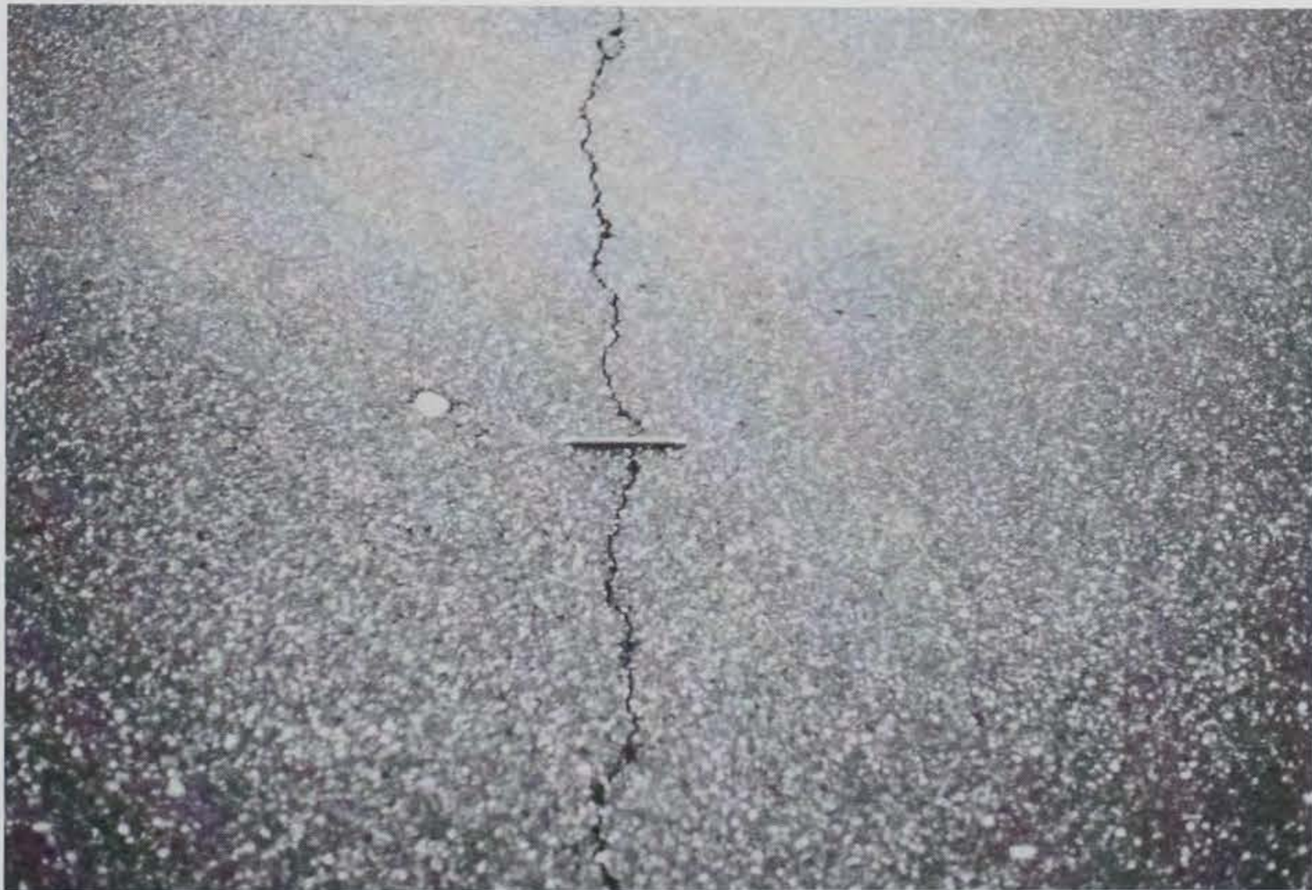
Figure 12. Asphalt-rubber section, US 98, McComb
