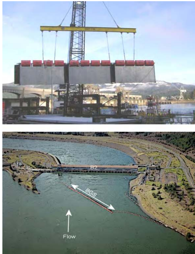
Figure 1.1. The Behavioral Guidance Structure with One Section Shown out of the Water (Top); and as Deployed in the Forebay of the Bonneville Dam Second Powerhouse (B2; Bottom)
