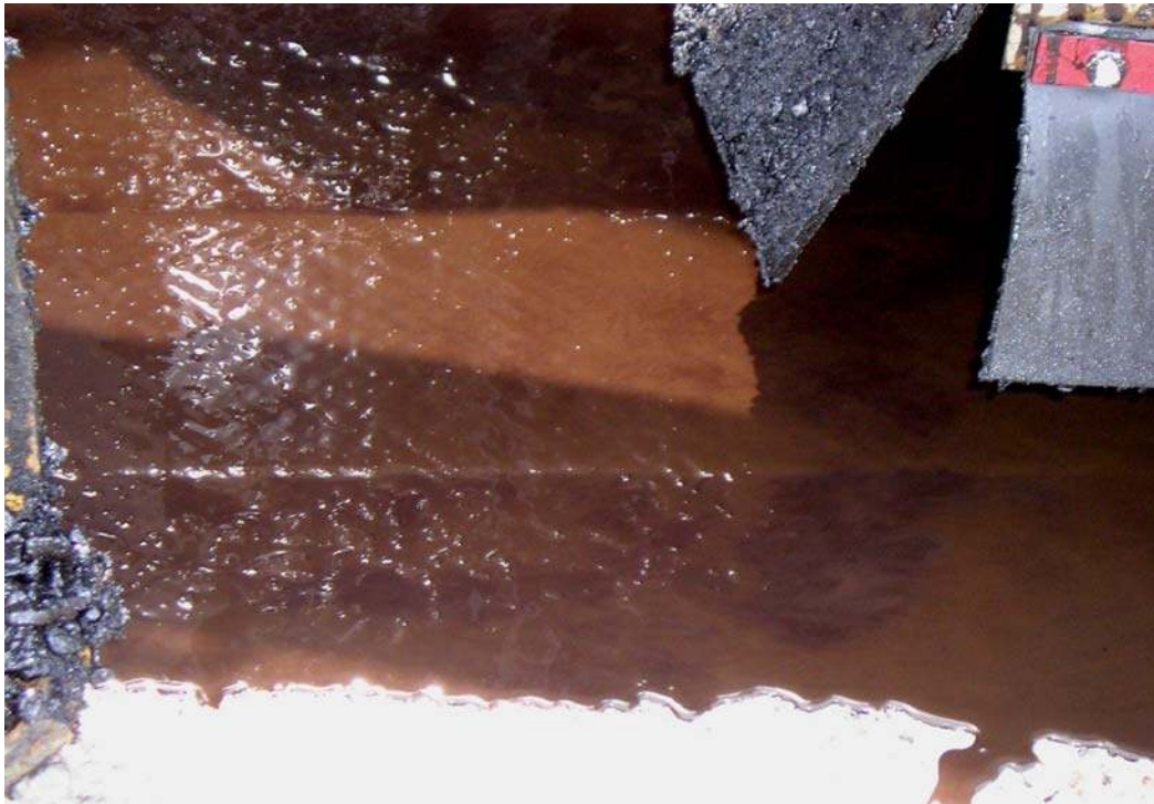
Figure 29. Tack Coat Applied by Novachip Spreader Just in Front of HMA
