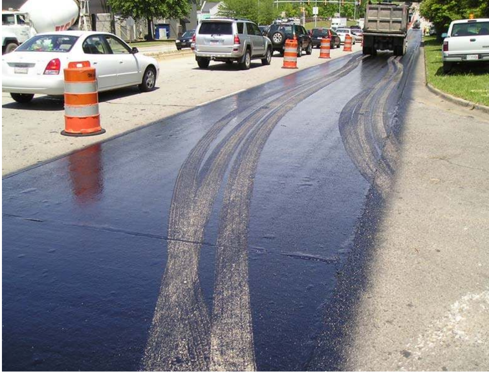
Figure 26. Tack Coat Applied with a Typical Distributor Truck on Project 6
