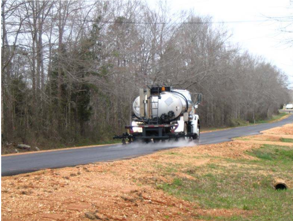
Figure 24. Application of CSS-1 Tack Coat on Project 5
