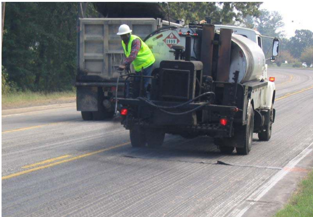
Figure 23. Application of Tack Coat with Hand Wand on Project 3
