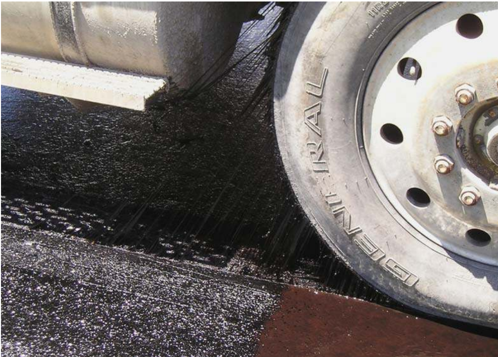
Figure 27. CQS-1HP Polymer Asphalt Emulsion as Applied in Section 1 & 2. Note the Strings of Tack Sticking to the Tire
