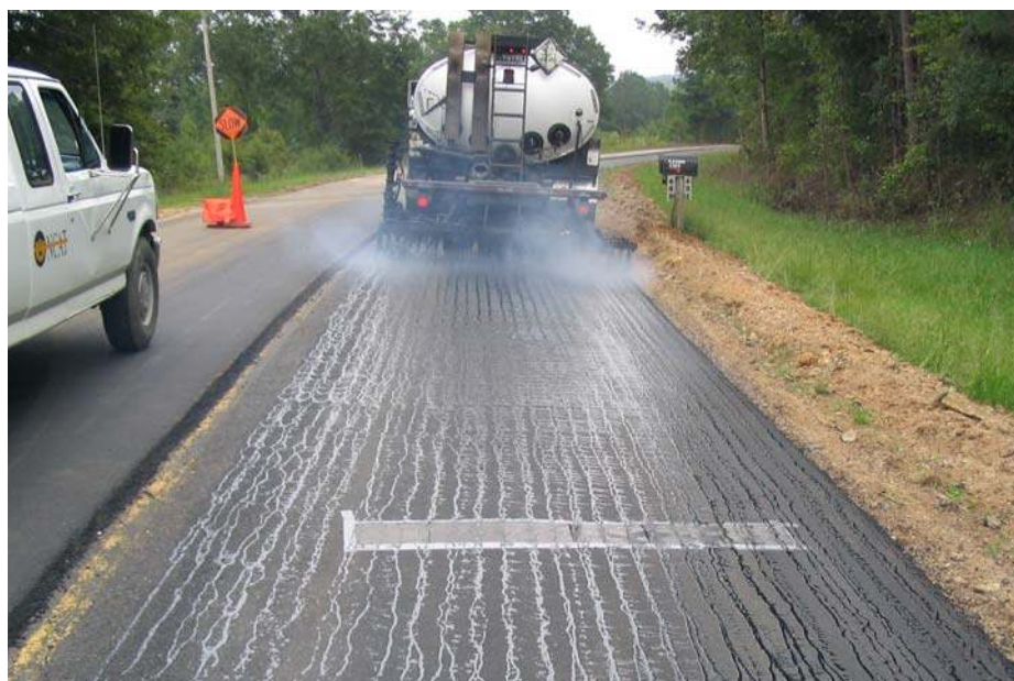
Figure 22. Application of PG 64-22 Tack Coat Test Section on Project 2
