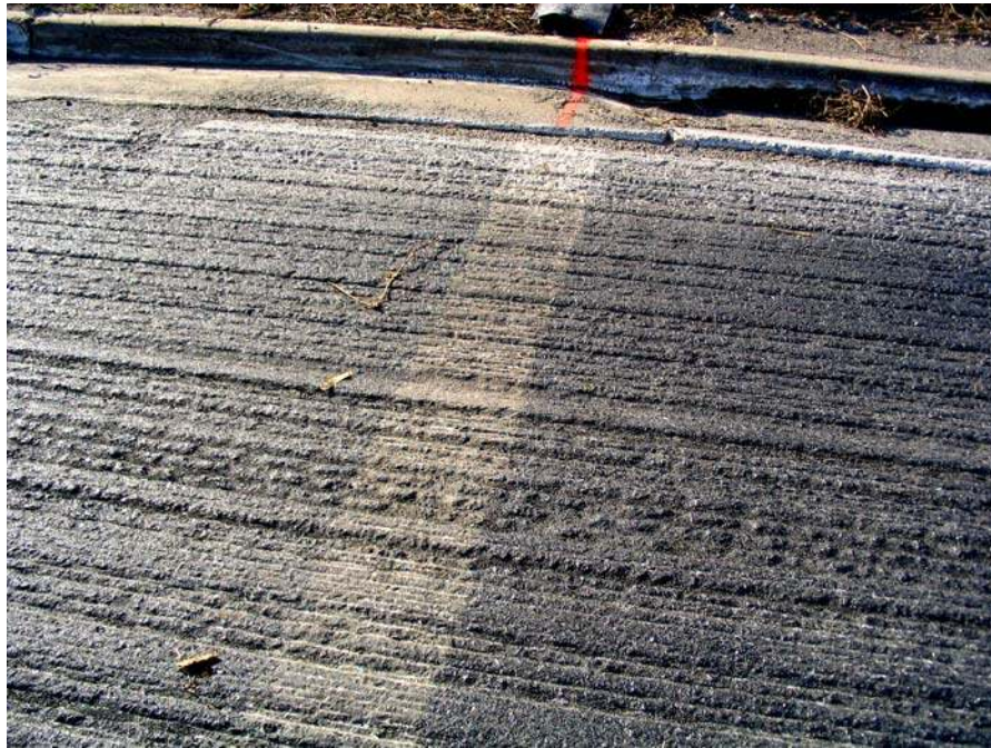
Figure 21. Photograph Showing Location Where Geotextile Pads Were Used to Measure Actual Tack Coat Application Rate
