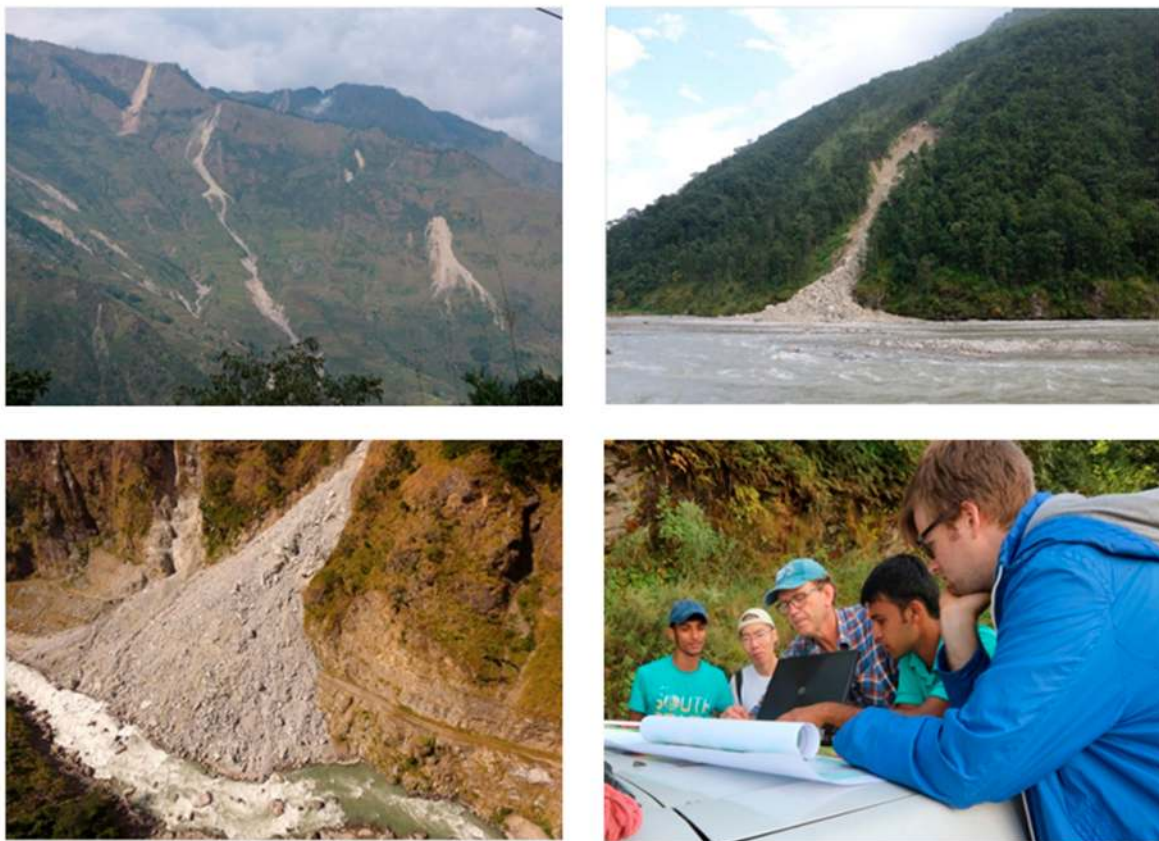
Figure 3. Field photographs showing landslide areas during field survey in the Rasuwa district.
