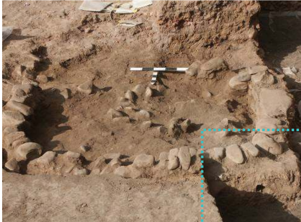
Figure 2.8: View of the Foundations (TAP 2006) Note original grade has been removed in the right hand corner to reveal foundations
