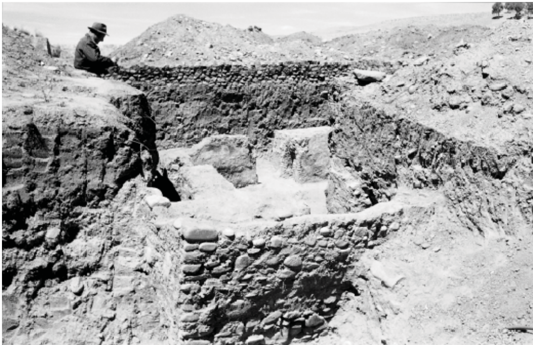
Figure 2.11: View of House One showing a general decay; no roofs; no drainage (Kidder Collection 1956)
