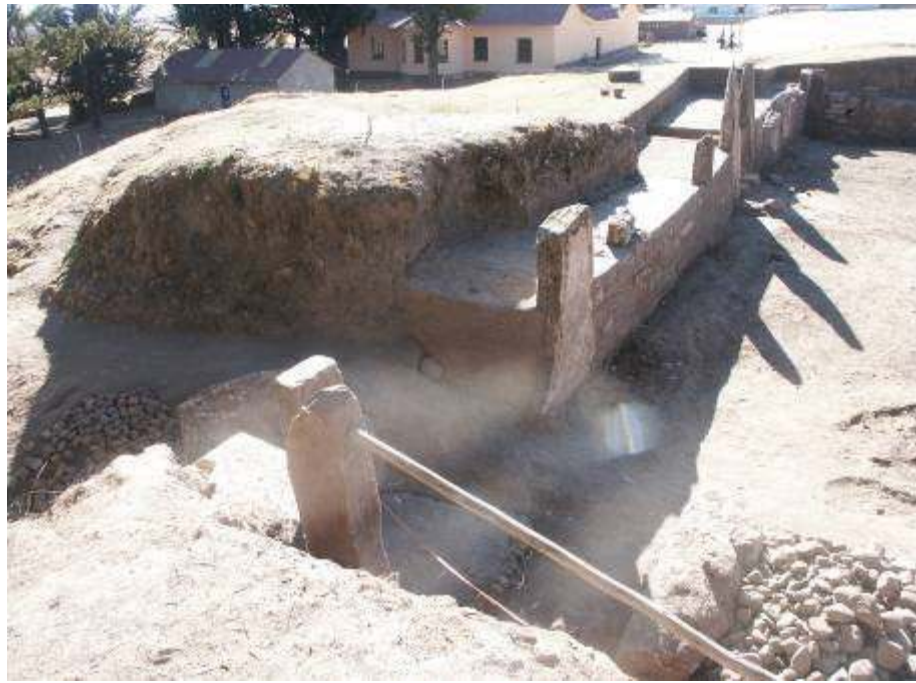
Figure 2.7: View of three-sided Tiahuanaco Platform under restoration (TAP 2006)
