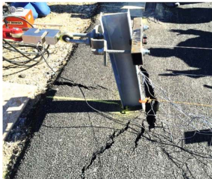
Figure 4. Asphalt rupture observed in the experimental program.
