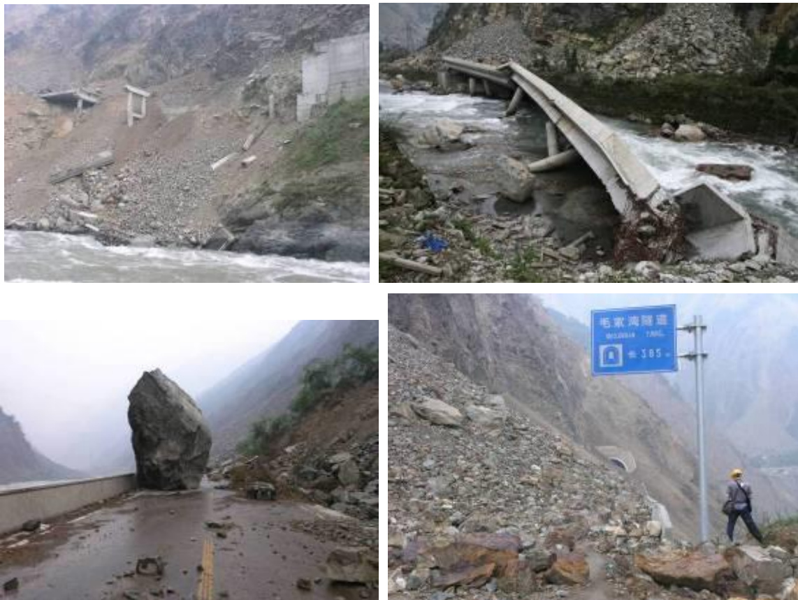
187 Fig. 2 Slope rock mass landslide in 5.12 Wenchuan earthquake destroys a bridge, blocks the road, buries smashes 188 tunnel entrance
