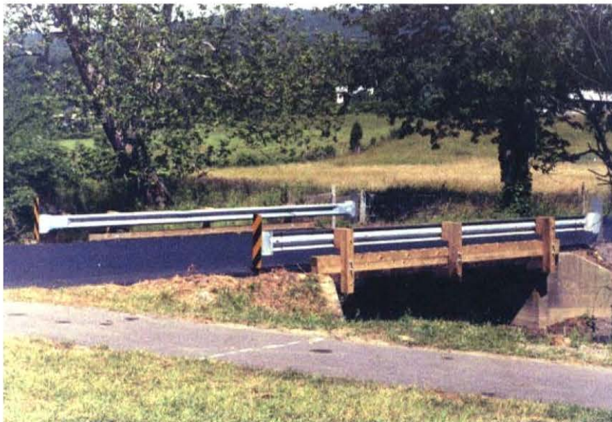
Figure 2. The completed Tom’s Creek Bridge.
