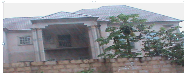
Figure 8. Contemporary duplex (ground floor) with stepped tiles and aluminum roofing sheets.
