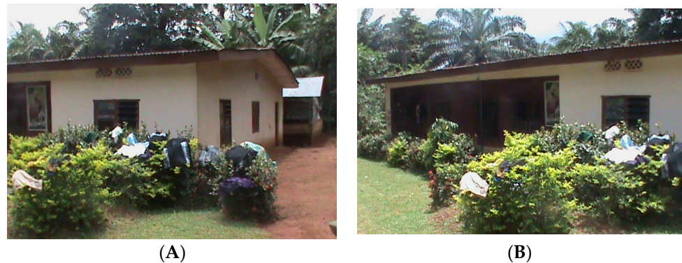
Figure 4. (A,B) A modern building with plastered and painted walls and corrugated iron roofing sheets.
