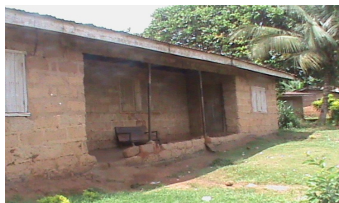
Figure 6. Contemporary bungalow with corrugated iron roofing sheets, unplastered and unpainted.
