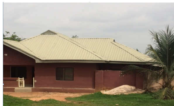
Figure 10. Contemporary bungalow with corrugated aluminum roofing sheets, plastered and painted.
