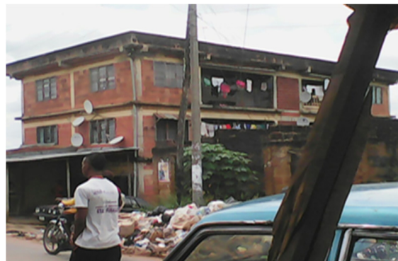
Figure 5. Contemporary structure with brick walls and corrugated aluminum roofing sheets.
