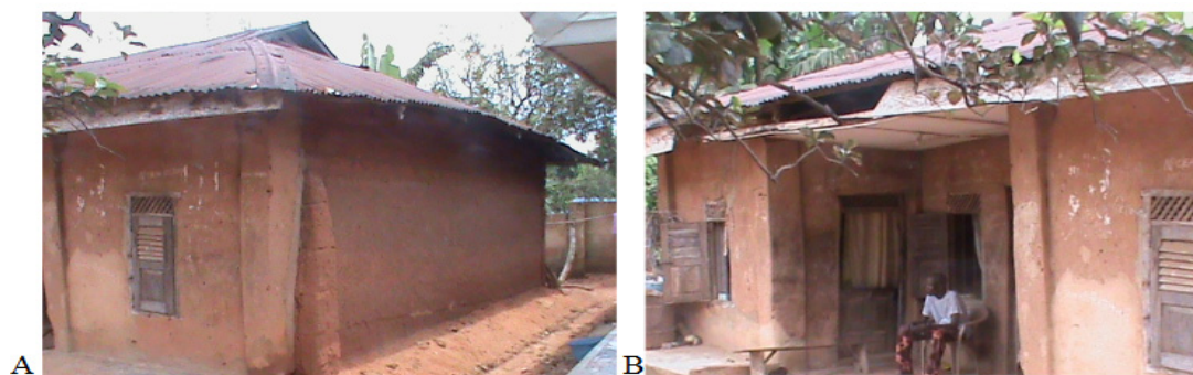
Figure 3. Traditional building (T2) with mud wall and corrugated roofing sheets (A,B).
