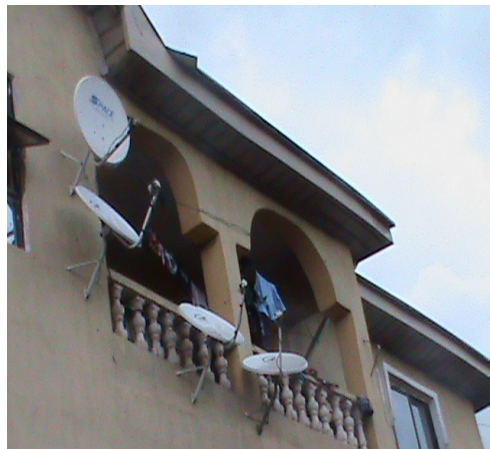
Figure 9. A modern structure with block walls and corrugated aluminum roofing sheets.
