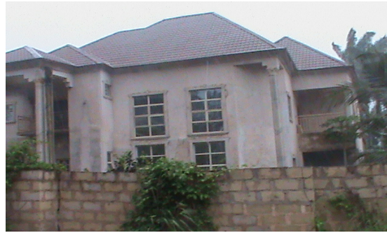
Figure 7. Duplex (top story) contemporary building with stepped aluminum roofing tiles.
