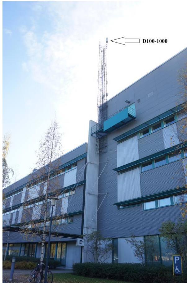
Fig. 3. The antenna is mounted on the University of Oulu antenna tower at a height of 24 m from sea level.
