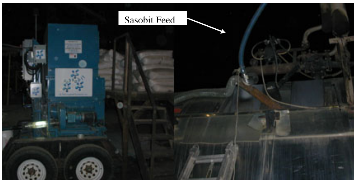
Figure 2. Sasobit® Pneumatic Feed to Mixing Chamber.
