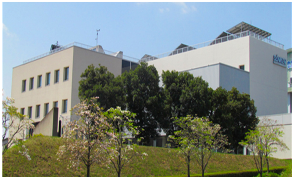
Figure 2. Photo of the target building.
