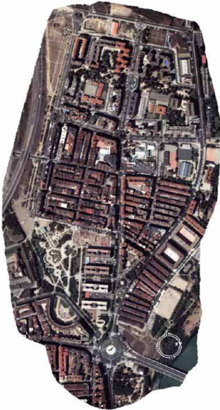
Fig. 4. Eye view of "La Almozara" in Saragossa (from Google Maps).
