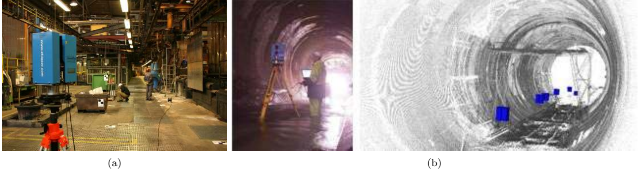
Figure 1: A 360°laser scanner of inmetris3D placed in a production hall (a) and in a tunnel with the resulting scan data (b). (All images courtesy of inmetris3D.)
