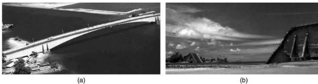
Fig. 1. (a) Koror-Babeldaob Bridge in Palau (in 1977); (b) Babeldaob side after the collapse (in 1996) (images courtesy DYWIDAG Systems International and Wiss, Janney, Elstner Associates, Inc., with permission)
