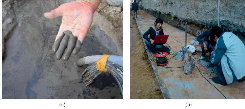
FIGURE 6: Test process. (a) Grouting. (b) Testing.
