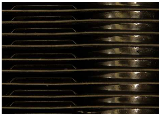
Figure 5 Front face of coil cleaned
