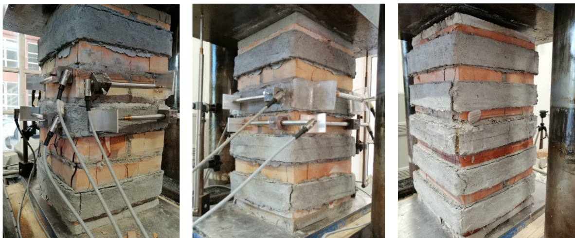
Figure 4. Partially confined columns at failure.
