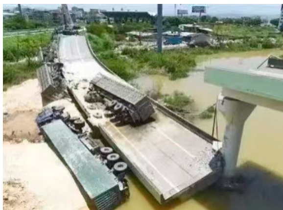
(b) Gane River source sluice bridge
