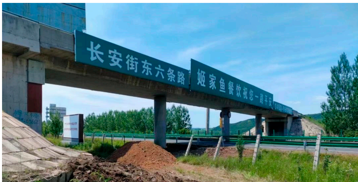
Figure 2. The real picture of separated overpass of the Hegang–Dalian Expressway.
