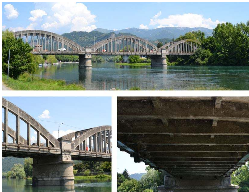
Figure 1: Contemporary views of Brivio bridge seen from Brivio's riverside (right bank).
