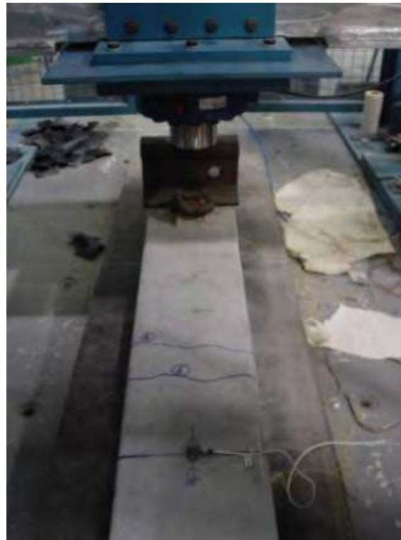
Figure 8.19 Cracks in a sleeper mid-span in soft track after 50 drops of 810 kN
