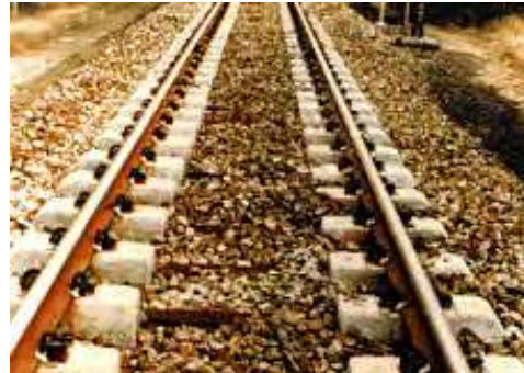
b) twin-block concrete sleeper
