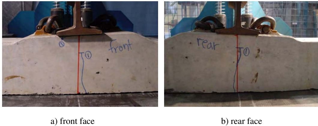
Figure 8.10 Cracks in a sleeper in hard track after a single impact of 740 kN
