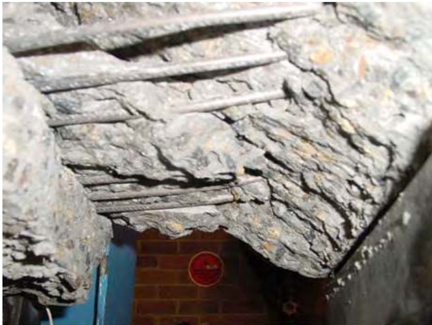
Figure 5.33 Prestressing wire inspection at rail seat
