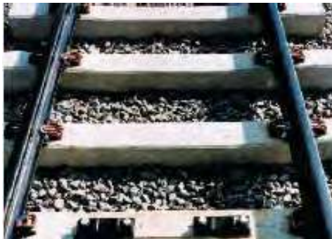
a) monoblock concrete sleeper
