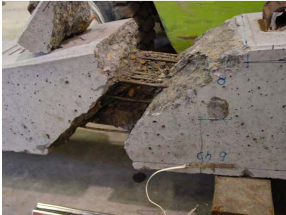
a) at applied-load rail seat
