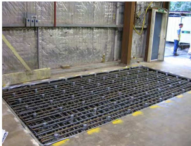
Figure 6.10 Steel frame for the strong floor
