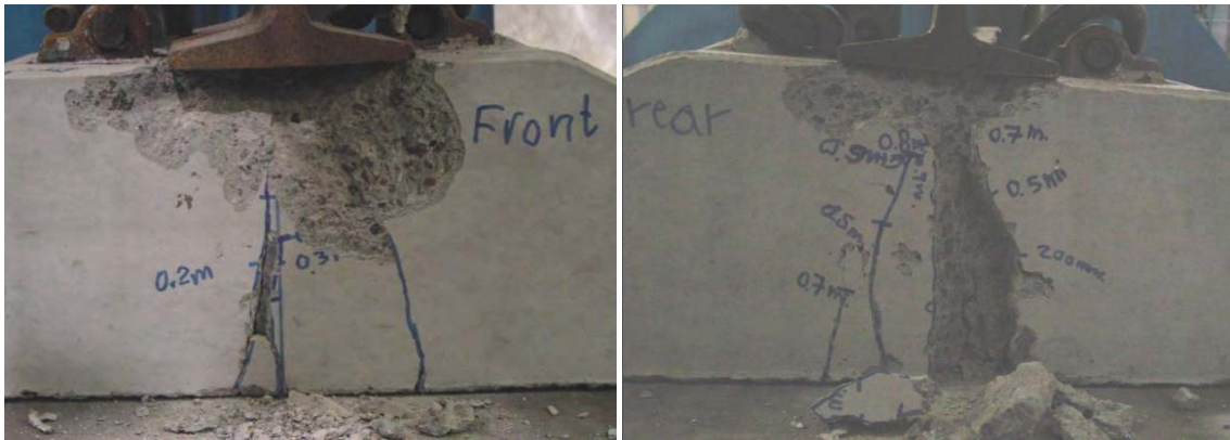
a) interfacial damage
