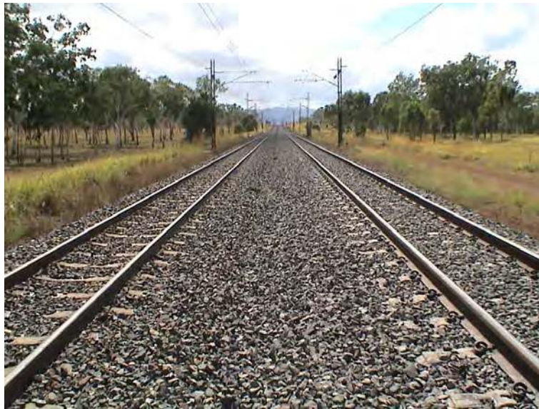
Figure 3.17. Typical ballasted track on a coal line in Central Queensland
