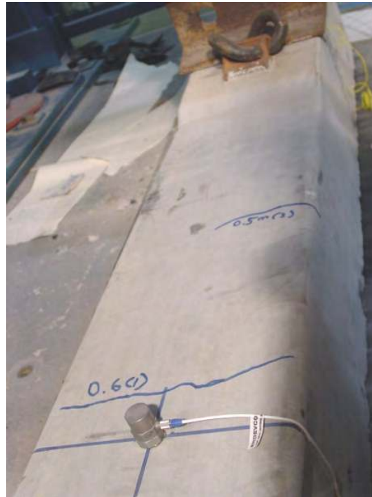
e) cracks on top surface
