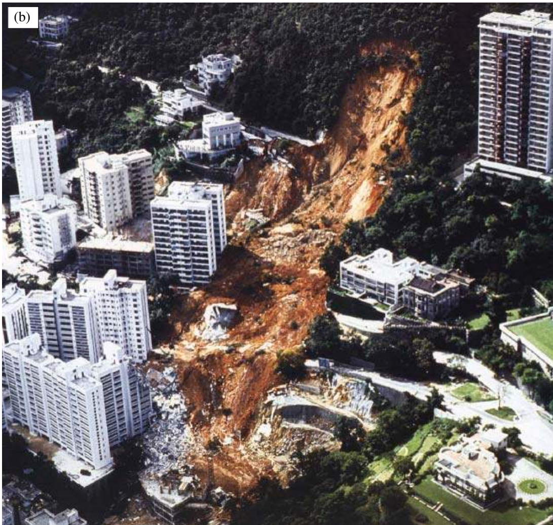
Figure 1.1 Two major slope failures in Hong Kong, 1972 - (a) Sau Mau Ping, Kowloon (b) Po Shan Road, Mid-levels
