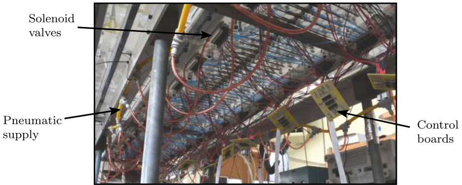
Fig. 10 A view of the underside of the actuated surface
