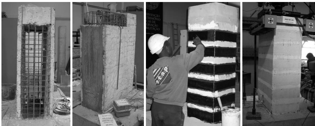
Figure 10: Hollow piers before and after the shear retrofitting with CFRP sheet
