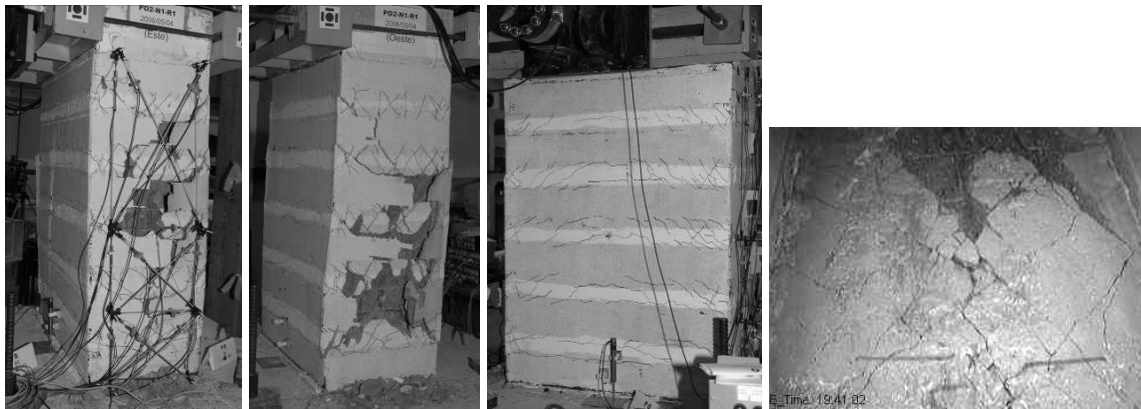
Figure 16: Final damage views of the retrofitted pier PO2 corresponding to 3.2% drift ratio.
