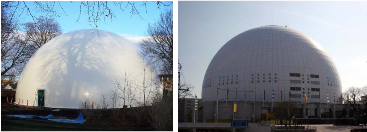
(a) Air inflated structure in Gentofte (Denmark) 1 . (b) Stockholm Globe Arena (by Tage Olsin CC BY-SA 2.0).
