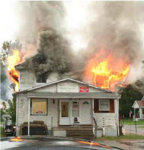
(a) Building fire
