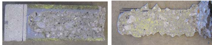
c. failure within concrete substrate (B-4 series)
