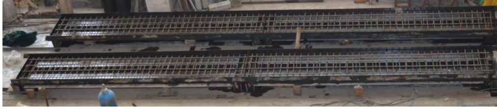
Fig. 3 Assembly of the form and arrangement of the rebar.
