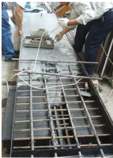
a Casting UHPC
