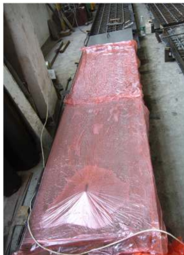
b Cover curing membrane
